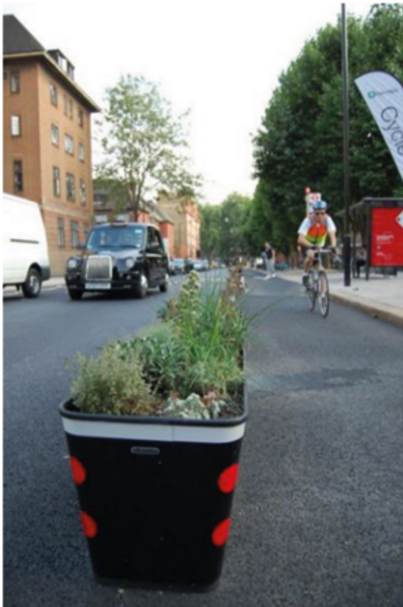
Figure 0.4: Planters segregating cycle lane, Camden
